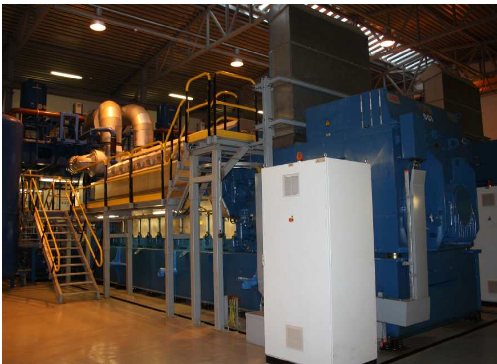
A section of the 24 Megawatt Diesel Generator-Set at Konkola
